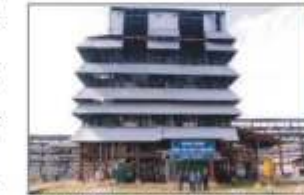
20,000 tpa plant established at Digboi for recovery of value added products from 'tank bottoms'
