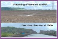
Flattening of Ulwe hill and Diversion of Ulwe river by Controlled Blasting Techniques implemented for construction of Navi Mumbai International Airport (NMIA) site.
