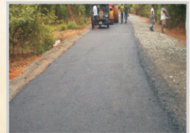
Cold mix laying and completion
