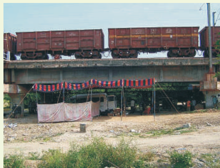
Fig. 1.44 View of the Railway Bridge
