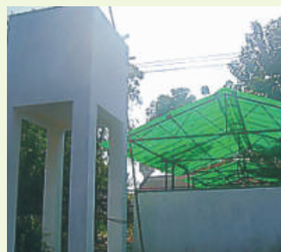
Ten ton Bioleaching Plant of Lateritic nickel ore
