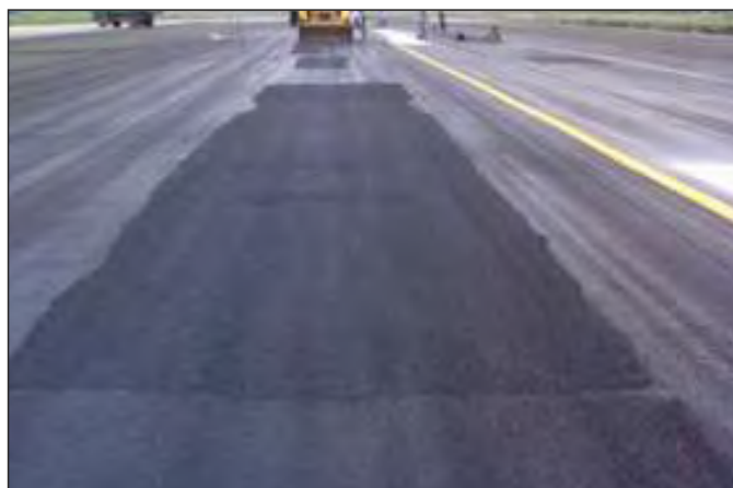
Fig. 1.49 Emergency Repair of Kolkata Runway
