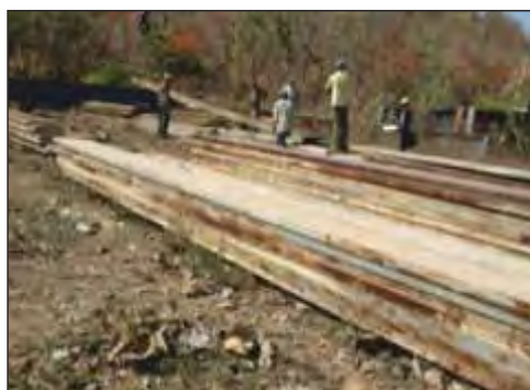
Fig: 1.38 Tie-flats of Sardar Sarovar Dam at storage site
