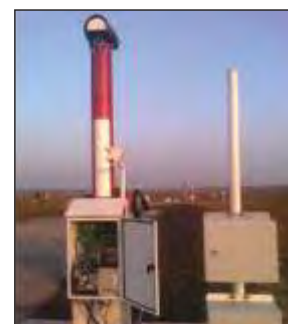
Fig: 1.59 Drishti at Main Runway 28-10 of IGI Airport
