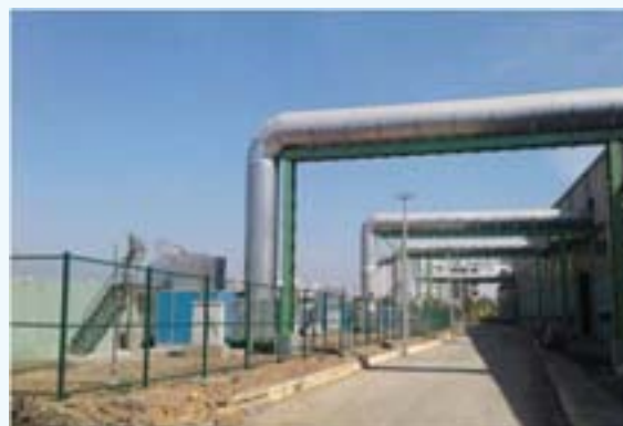
Fig: 7.8 Odour control system at 500 tpd MSW mechanical biological treatment plant at KCDC, Bengaluru. Exhaust ducting from plant (on the right) to biofilters (on the left).
