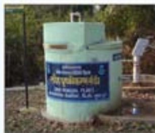
Fig:7.18 Hand pump attached iron removal plant
