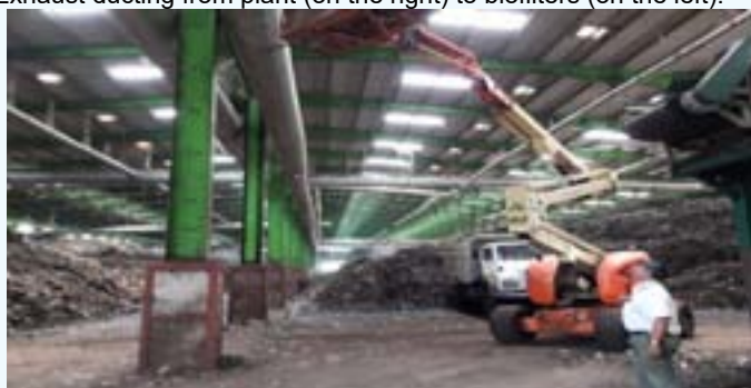
Fig: 7.9 Gas biofilters under construction at 500 tpd municipal solid waste treatment facility. Installation of exhaust ducting.
