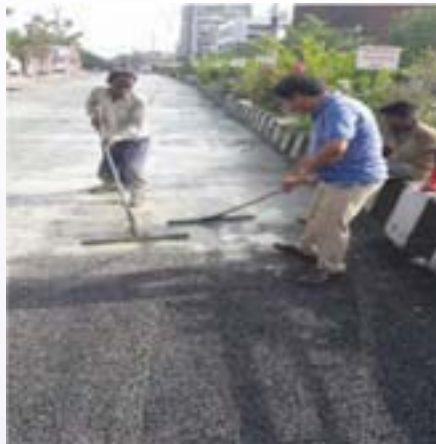
Fig. 8.3.11. View of pouring of grout and squeezing on high voids bituminous mix
