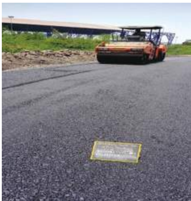
(c) Laying of DBM using Steel
