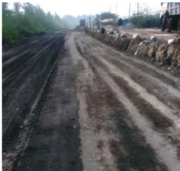
(b) Laying of Granular Sub-Base using Steel slag
