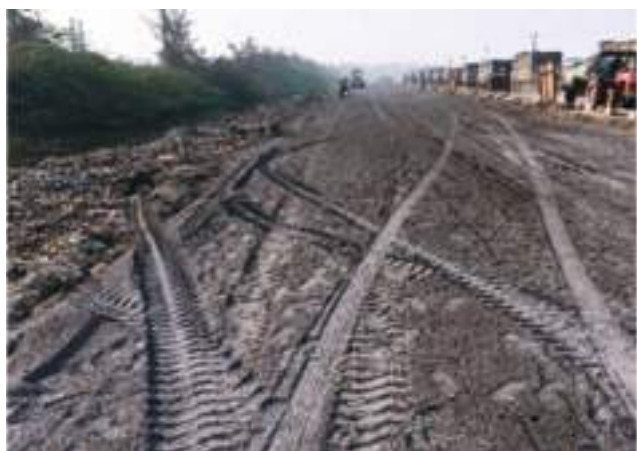
(a) Steel Slag Sub-grade
