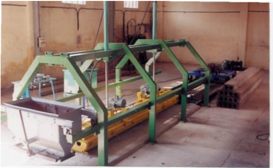
Mechanised casting of concrete Cored Unit
