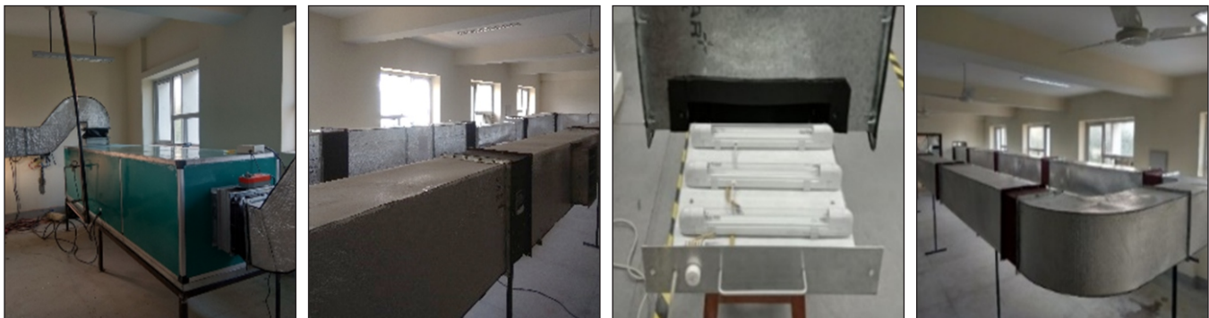
Figure 18: Photos of the Test Bed Facility on Technology Testing and Evaluation (TTE TBF ) at CSIR-CBRI, Roorkee
