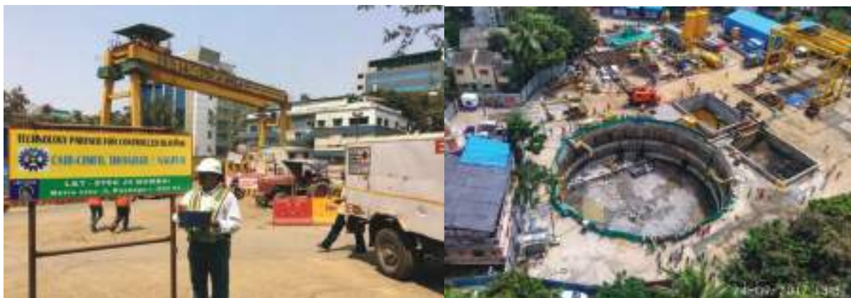
Fig. 7.25: Controlled blasting technology for construction of Bangalore and Mumbai Metro Rail Projects
