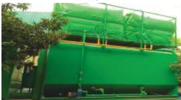
Fig. 6.2.5: Full scale biogas plant for the treatment of food waste at Capgemini, Hyderabad
