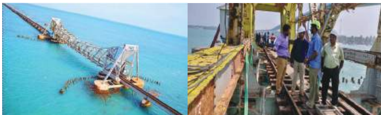
Fig. 7.23: Structural integrity assessment of the Scherzer span of the Pamban railway bridge
