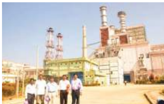
Fig. 7.15: Reactor containment building at Kalpakkam
