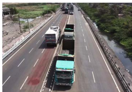
Aerial view of Steel Slag Road built at Hazira, Surat
