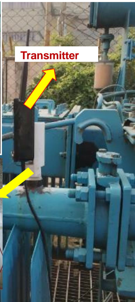
On-site installation of low ppm moisture sensor and digital meter for online measurement of moisture in transformer oil
