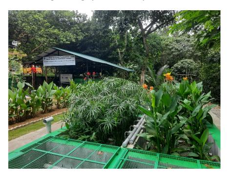
The NOWA integrated Bio-Eco engineering system is developed for treating and reusing household greywater. Compared with existing technologies this system requires less (30-40%) space and it can handle high strength greywater. Presently one 10 KLD unis is operational in NIIST campus treating the NIIST staff quarters greywater and reusing the treated water for gardening and agriculture in NIIST campus.
