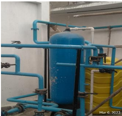
Multigrade Filter, and sludge Drying Reed Beds
