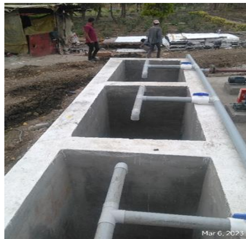
Multigrade Filter, and sludge Drying Reed Beds
