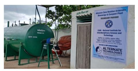
Based on CSIR-NIIST solid state bio-methanation technology, a model treatment system for treating ~250 kg farm waste into biogas was setup in the Durg district of Chhattisgarh. The biogas produced was supplied to a nearby govt. school for preparing mid-day meals for school kids
