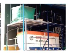
NOWA (NIIST onsite wastewater treatment system) is modular onsite wastewater treatment and resource recovery unit. This is a patented technology, and this technology is approved by Kerala state Suchitwa mission for field implementation. Already 4 companies licensed this technology, and field units up to 10 KLD are working at different industrial site
