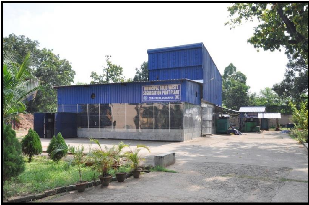
Integrated Solid Waste Management Plant at CSIR-CMERI Durgapur
