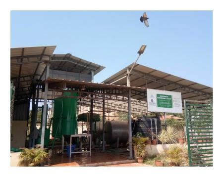
The entire food waste in both domestic and international terminal is treated in this system, which is compact and operates with minimal water requirement, and produces more biogas. The biogas produced is recovered as electricity.
