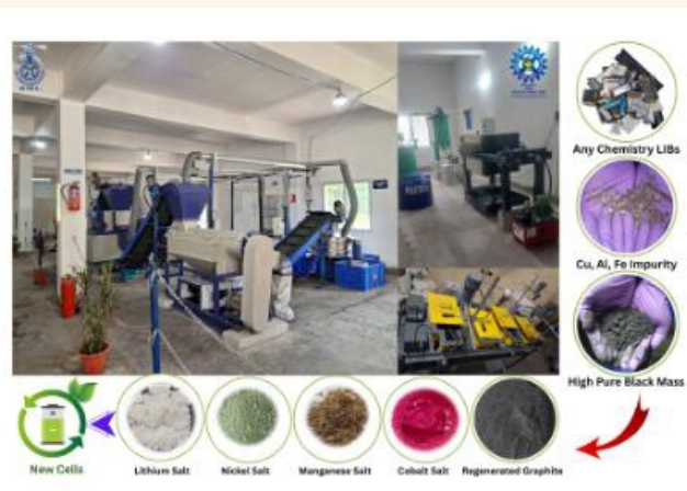
Battery Recycling Pilot Facility, Jamshedpur
