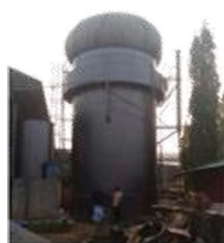
BFBR with double membrane gas holder. Licensee: Galaxy Environ Pvt. Ltd.
