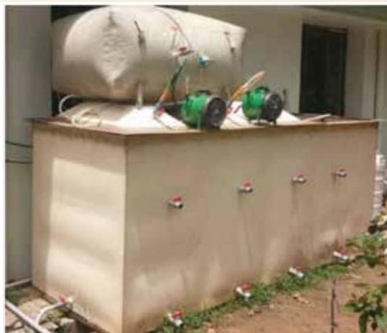
NOWA unit (2000L/day) installed in NIIST campus recovering biogas and reuse quality water from high strength wastewater discharged from NIIST canteen
