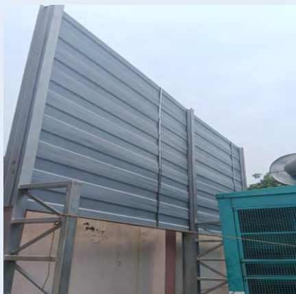
Field installations of the frequency based noise barrier on the DMRC network, New Delhi, and B. R. Ambedkar Road, Mumbai.
